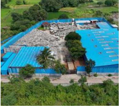
Sankalp’s 2023-established Hinjawadi aluminium formwork factory drives faster construction across all projects.
