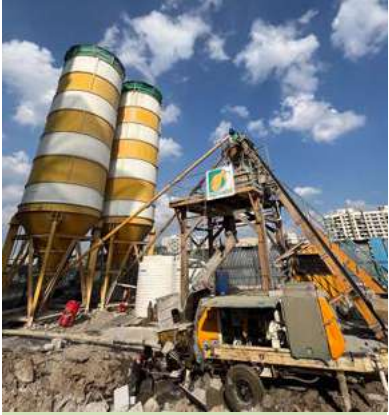
With an annual output of over 3 lakh cubic metres of concrete, Sankalp deliver at least one slab every day across their Pune locations.
